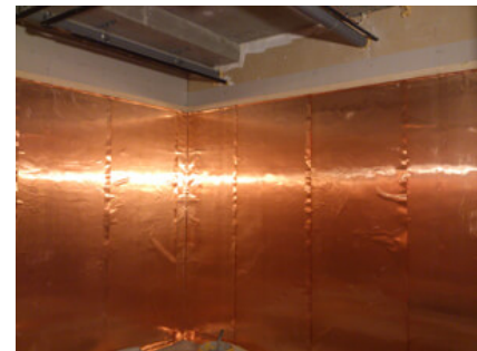
MRI room covered with Mu-copper foil before it is covered with plaster board or other desired finish
